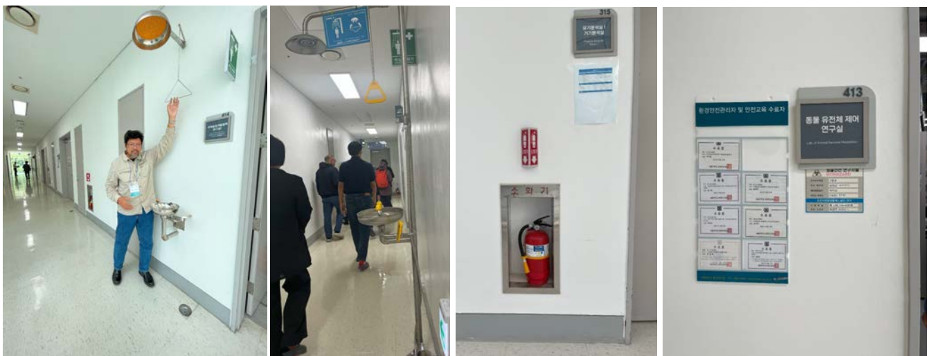
Emergency shower and fire extinguishers in Laboratory and permission for research workers
